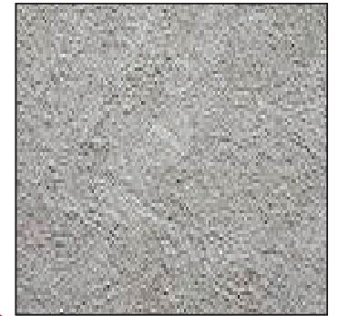
GRAY STUCCO LOCATED AT ROOFTOP PATIOS
