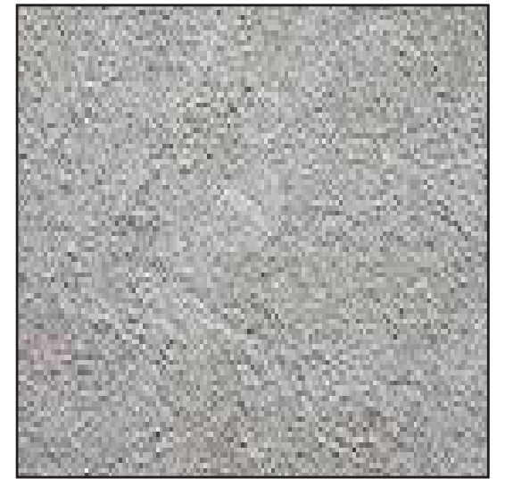
GRAY STUCCO LOCATED AT ROOFTOP PATIOS
