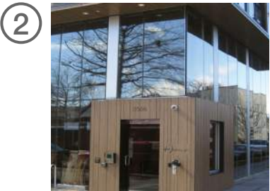
② Butt-glazed storefront allows for seamless glass wrap
