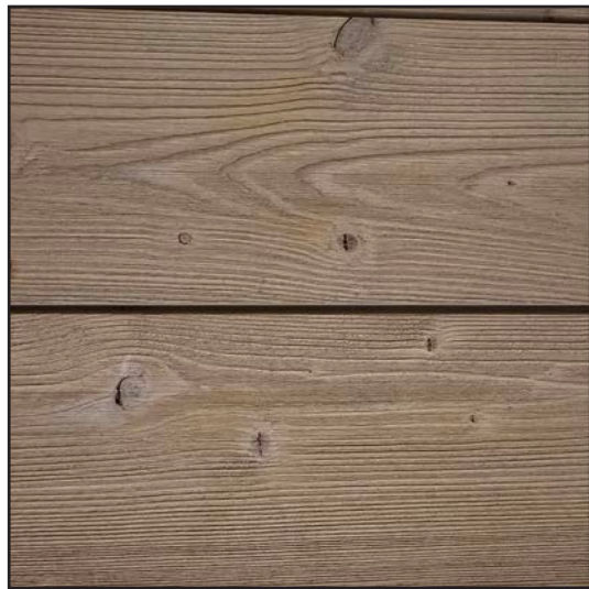
STAINED CEDAR WOOD SIDING
