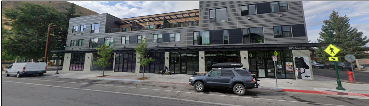
Figure 1. Curb face site view
