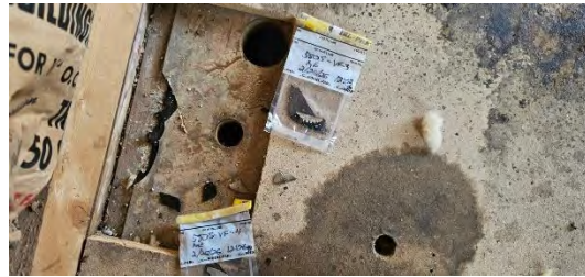
VINYL SHEET FLOORING UNDER EXPOSED PARTICLE BOARD SUBFLOOR IN MIDDLE ROOM
