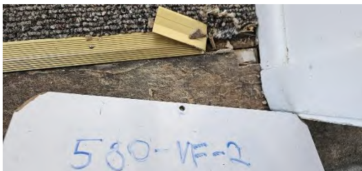
VINYL/LAMINATE FLOORING IN LAUNDRY ROOM
