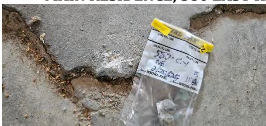
CONCRETE SLAB ON GRADE IN GARAGE
