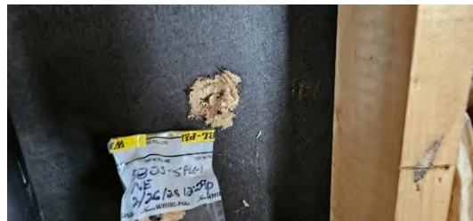
FIBERBOARD SHEATHING UNDERLYING SIDING ON NORTH HALF OF STRUCTURE
