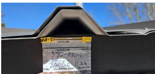
FELT UNDERLYING METAL ROOFING
