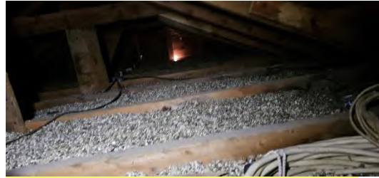
VERMICULITE INSULATION (VERM-2) ABOVE CEILING OF SOUTH ROOM (<0.25% ACTINOLITE/TREMOLITE ASBESTOS)
