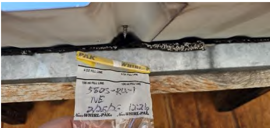
OLDER ASPHALT SHINGLE ROOFING, BLACK TAR, AND FELT UNDERLYING MEAL ROOF (8% CHRYSOTILE ASBESTOS IN BLACK TAR)
