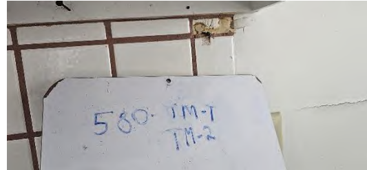
TILE AND MORTAR BACKSPLASH IN KITCHEN
