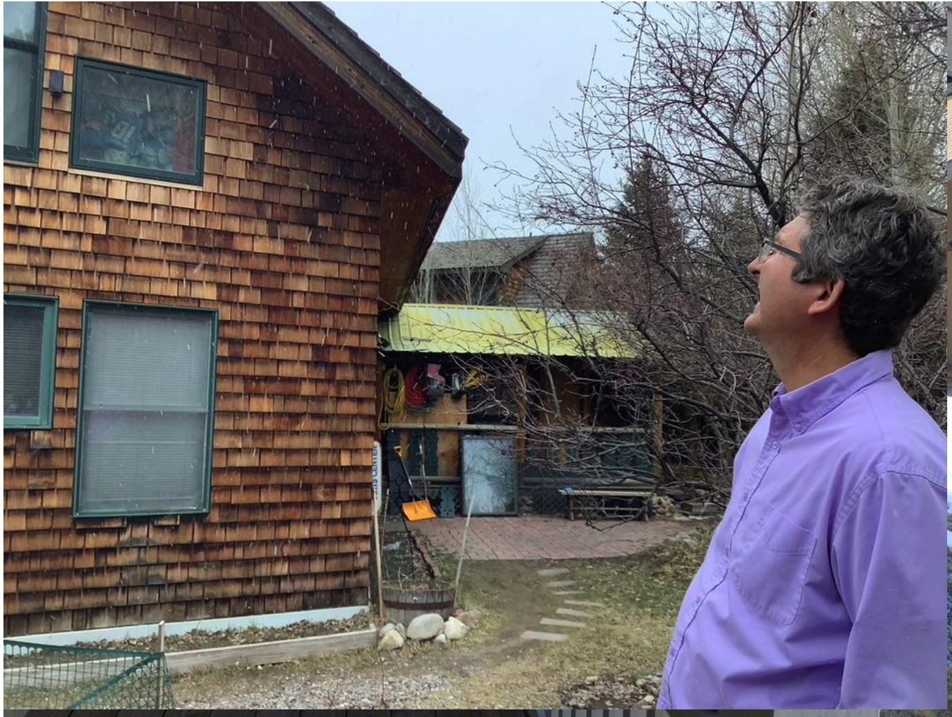
PHOTO #5 - (E) CABIN ADDITION #2 TO BE DEMOLISHED AND ITS CONTEXT WITH EXISTING HOUSE.
