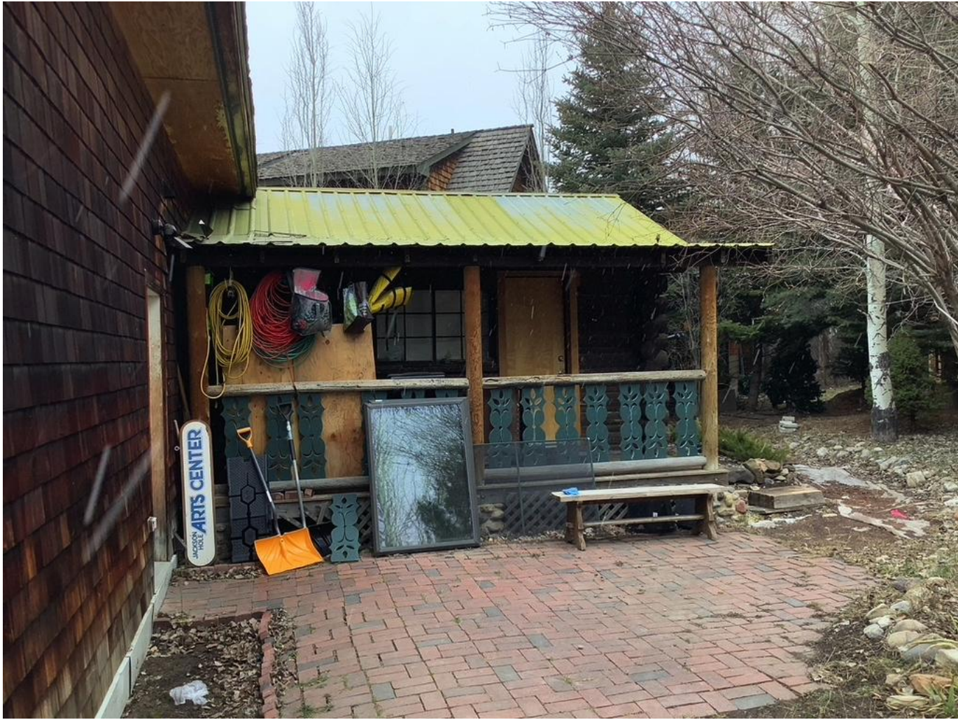
PHOTO #6 - (E) CABIN ADDITION #2 CLOSE UP VIEW #1
