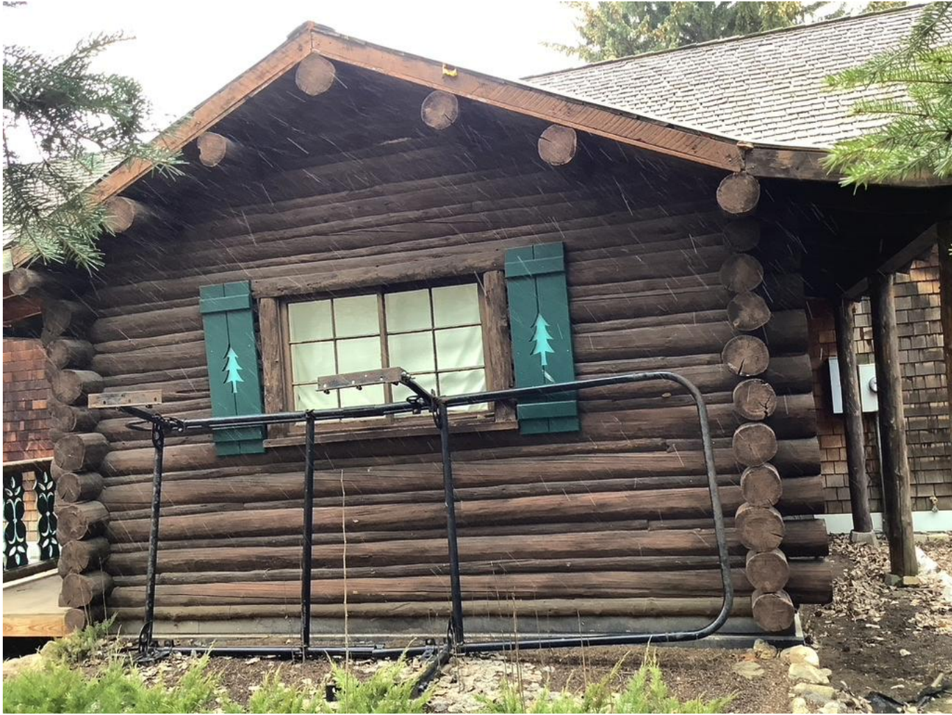
PHOTO #7 - (E) CABIN ADDITION #2 CLOSE UP VIEW #2
