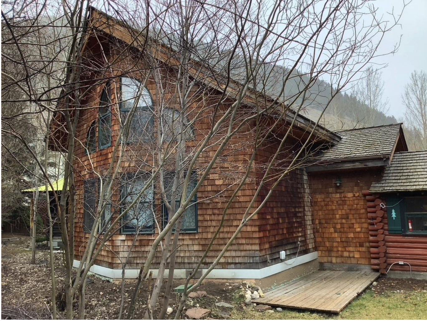
PHOTO #3 - EXISTING CABIN #1 ADDITION & CONNECTOR IN CONTEXT ON HOW IT CONNECTS TO EXISTING HOUSE TO REMAIN.
