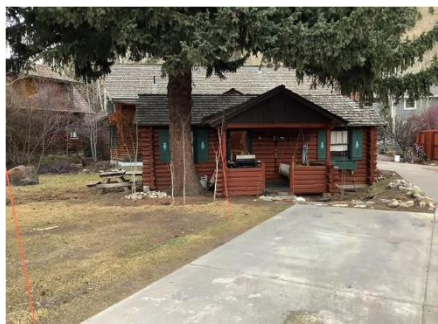
EXISTING CABIN #1 ADDITION TO BE DEMOLISHED W/ CONCRETE DRIVEWAY IN BACKGROUND TO ALSO BE DEMOLISHED
