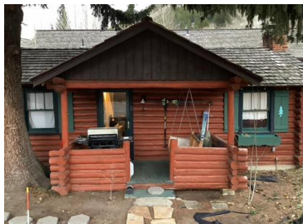
EXISTING CABIN #1 ADDITION FRONT ENTRY VIEW.
