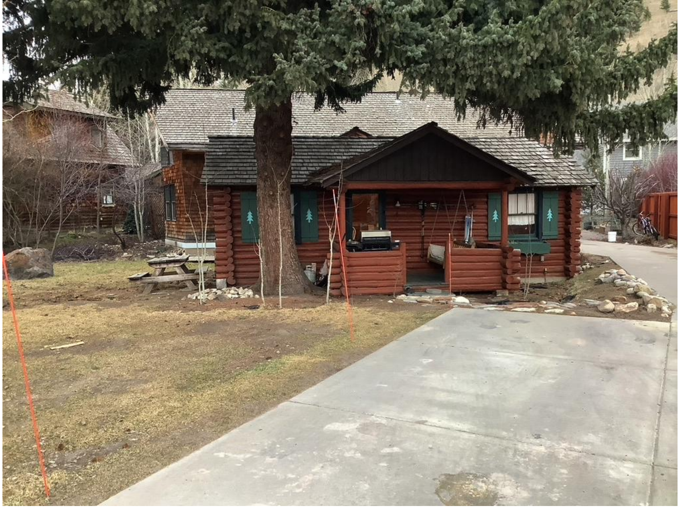
PHOTO #1 - EXISTING CABIN #1 ADDITION TO BE DEMOLISHED W/ CONCRETE DRIVEWAY IN BACKGROUND TO ALSO BE DEMOLISHED.
