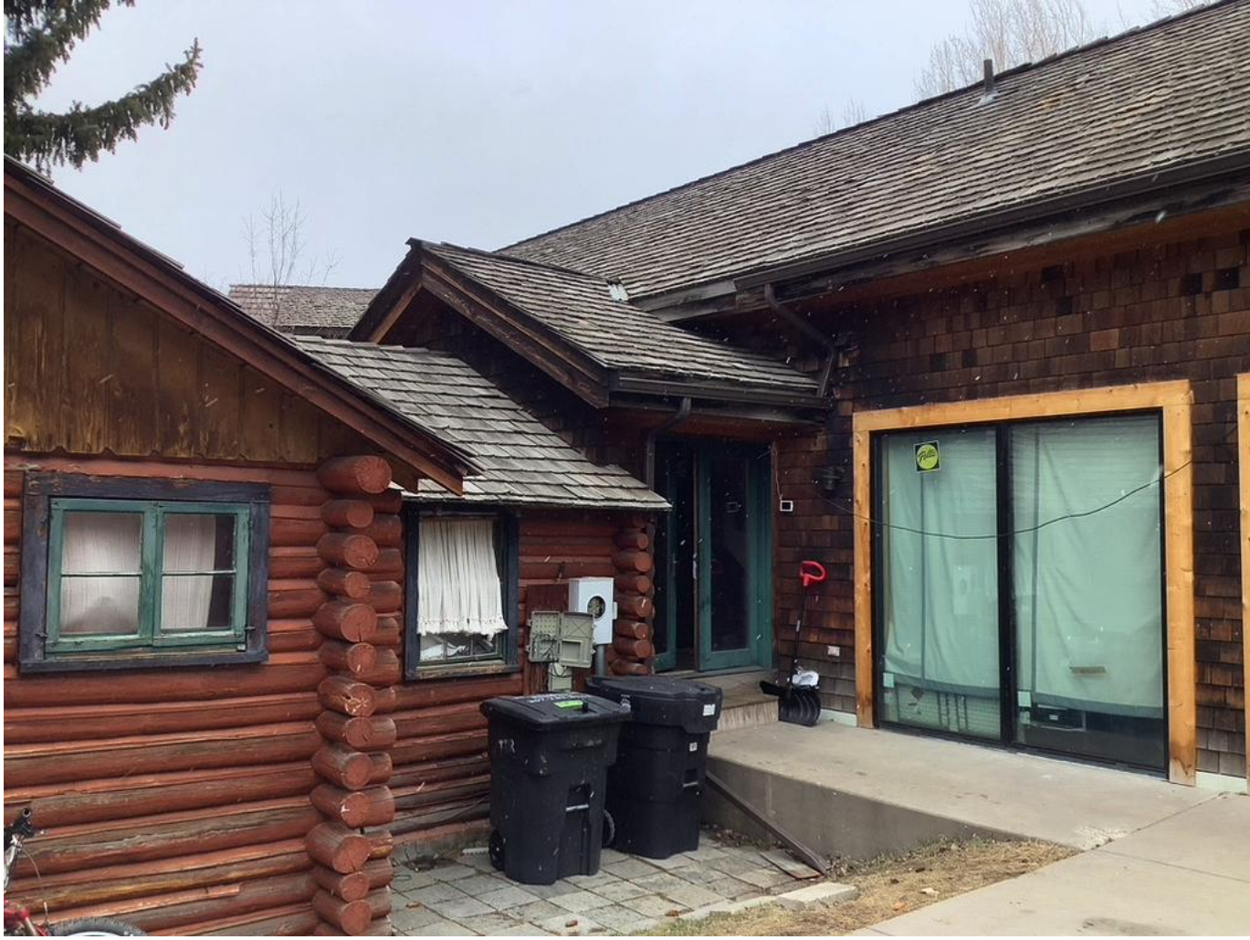
PHOTO #4 - EXISTING CABIN #1 ADDITION & CONNECTOR IN CONTEXT ON HOW IT CONNECTS TO EXISTING HOUSE ON OPPOSITE SIDE.
