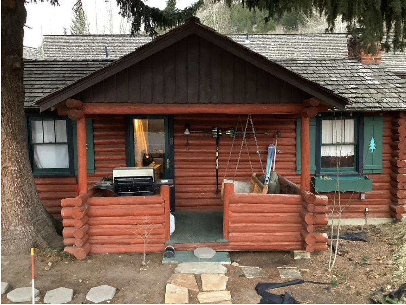
PHOTO #2 - EXISTING CABIN #1 ADDITION FRONT ENTRY VIEW
