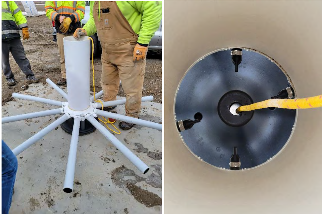
Figure 6: Combined Coarse-Bubble and Fine-Bubble Diffuser Assembly (Tiplepoint)
