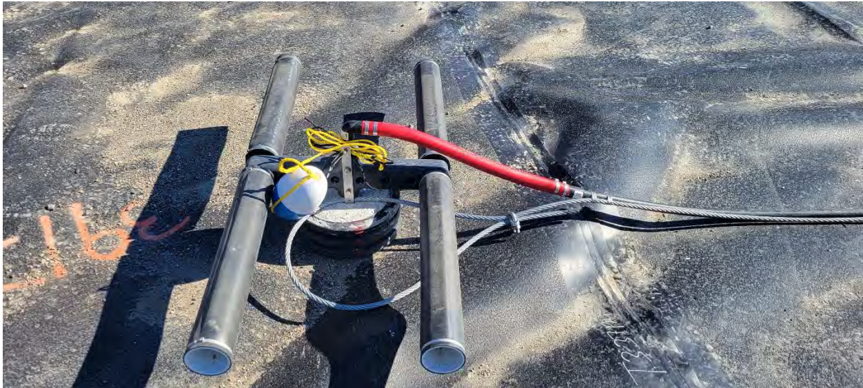
Figure 5: Fine-Bubble Diffuser Assembly
