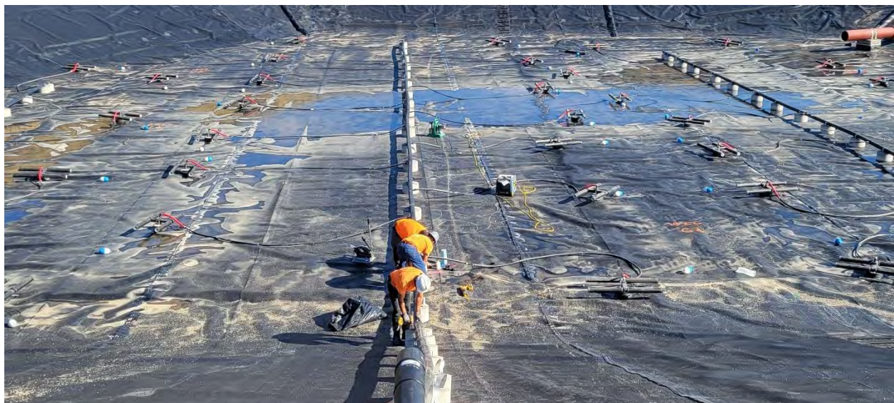
Figure 2: Submerged Laterals with Diffusers Sitting on Bottom
