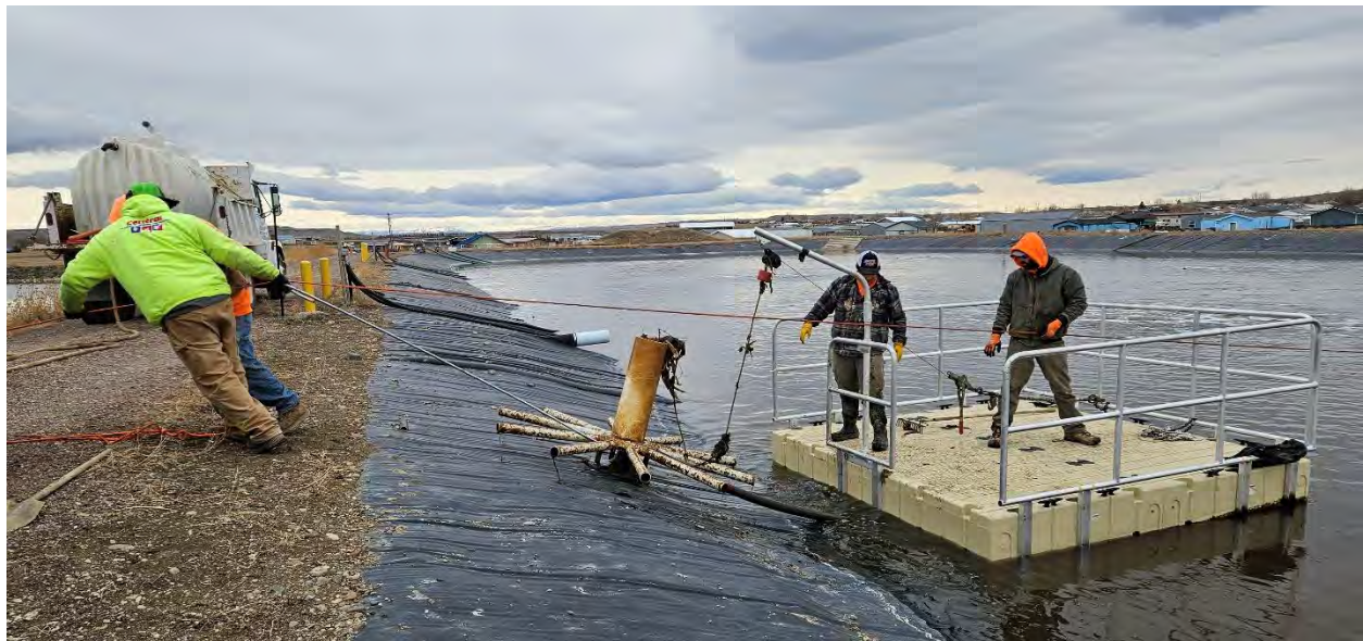
Figure 4: Maintenance on Diffuser Assembly with Individual Feeder Tube
