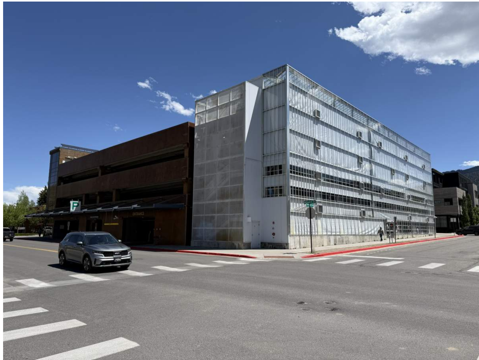
VERTICAL HARVEST / PARKING STRUCTURE 160 SOUTH MILLWARD
