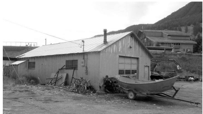
Figure 13: Maintenance shop (Mary Humstone, 2011)
