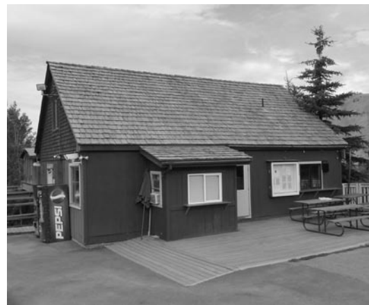
Figure 16: Rafferty lift building (Mary Humstone, 2011)
